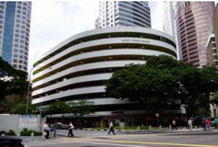
The old facade
