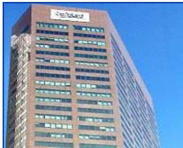
Six Battery Road
