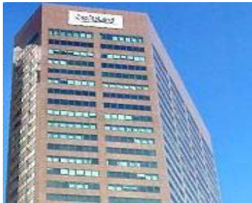
Six Battery Road
