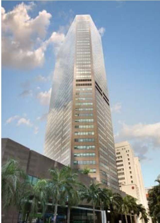
Six Battery Road
