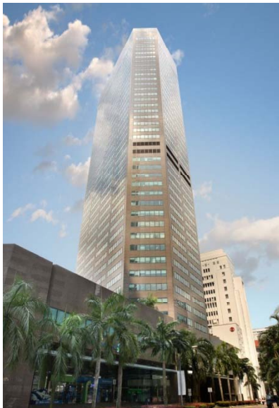
Six Battery Road
