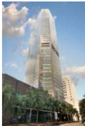
Six Battery Road
