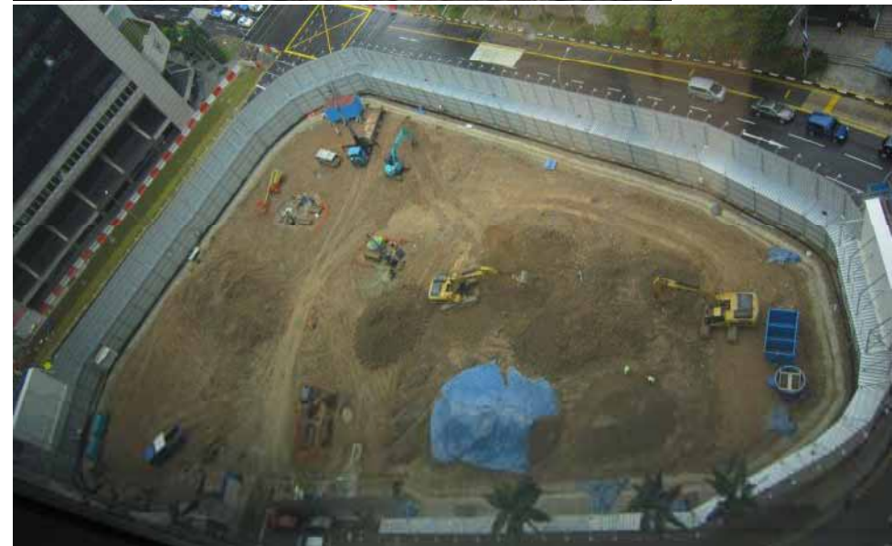
December 2011 – Demolition works completed
