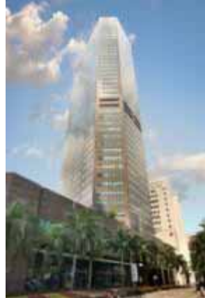
Six Battery Road
