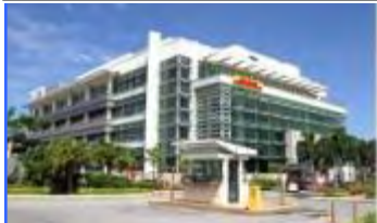
Quill Building 4 - DHL 2
