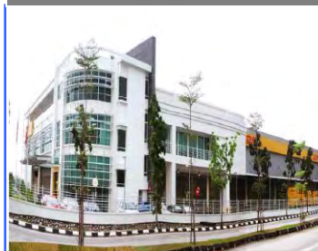
Quill Building 8 - DHL (XPJ)
