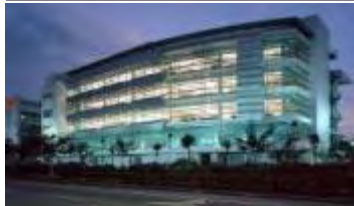
Quill Building 1 - DHL 1
