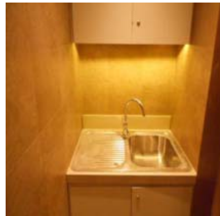
Addition of wet pantry for tenants' convenience
