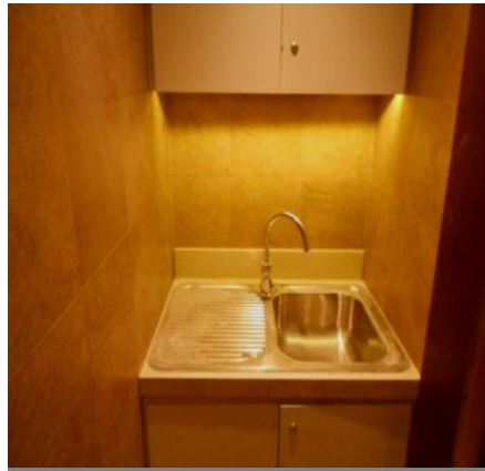
Addition of wet pantry for tenants' convenience
