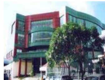
Quill Building 10 - Section 13
