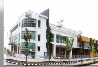
Quill Building 8 - DHL (XPJ)
