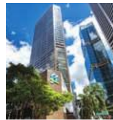
5 SIX BATTERY ROAD
