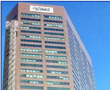
Six Battery Road
