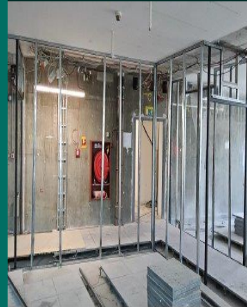
Drywall partition works
