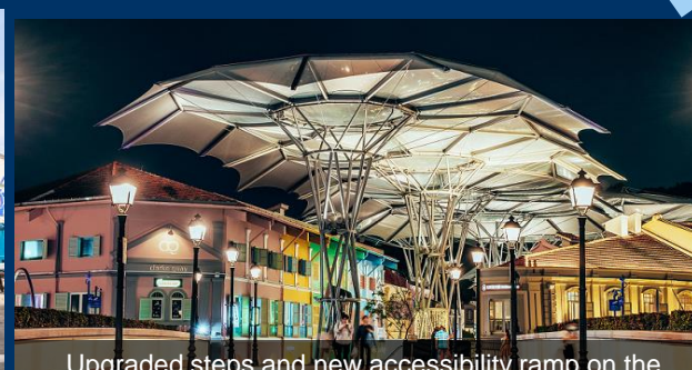
Upgraded steps and new accessibility ramp on the Read Bridge and improved thermal comfort along the internal streets
