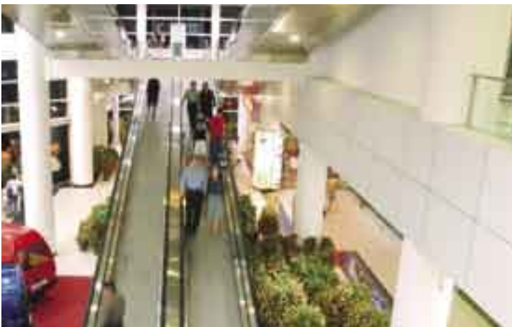
Newly installed travellators
