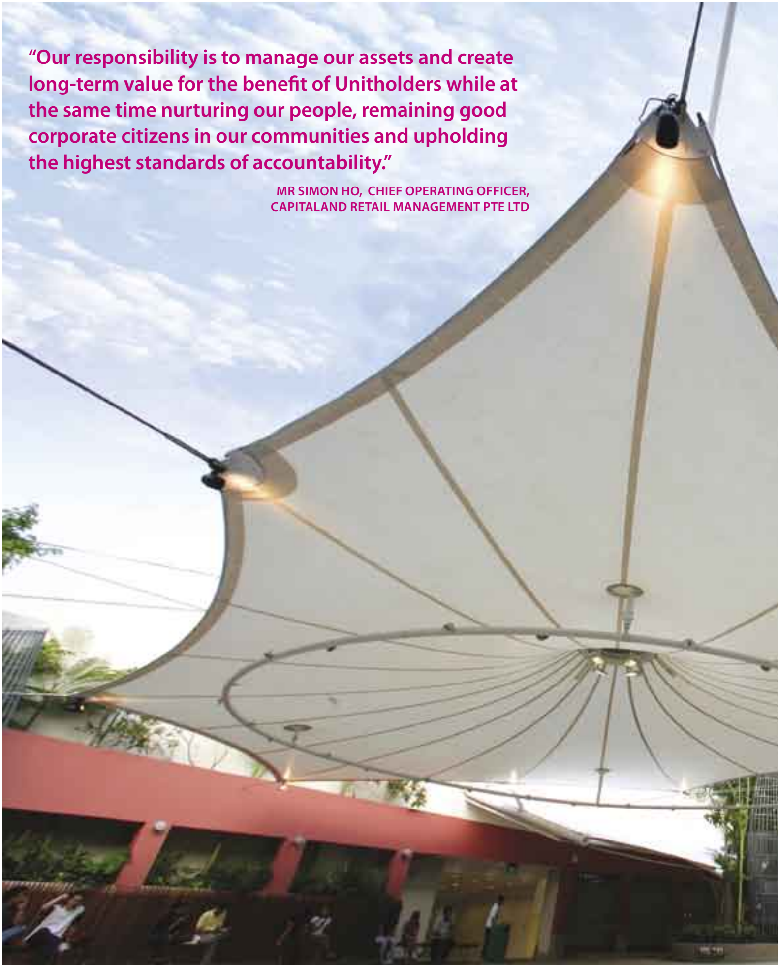
Rooftop landscape plaza at Tampines Mall
