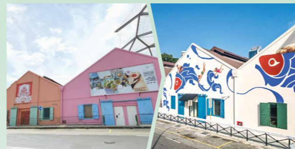
▲ Restored Block B's façade featuring a mural artwork which takes reference from Clarke Quay's heritage as a Teochew enclave
