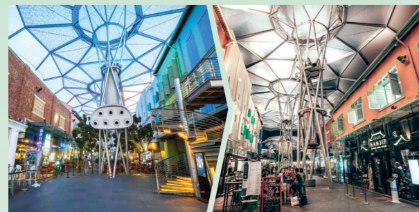
▲ Angel canopies with improved Ethylene Tetrafluoroethylene (ETFE) membrane and new omni-directional fans lower environmental temperature
