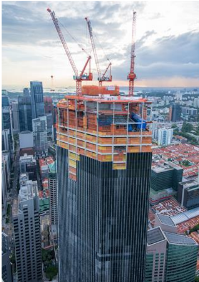
CapitaSpring topping-out at level 51
