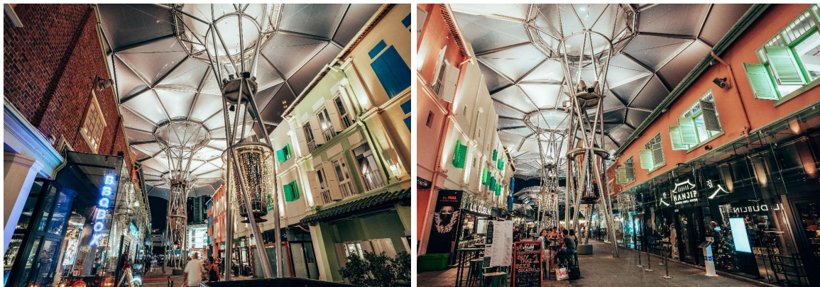
Angel Canopy along the internal streets with improved ETFE membrane
